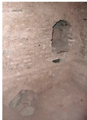
Fig. 7 Ceiling and walls are covered with Tadelakt, a special lime plaster
