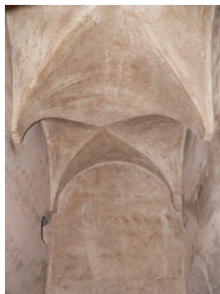
Fig. 7 Ceiling and walls are covered with Tadelakt, a special lime plaster
