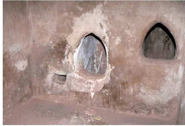
Fig. 11+12 Different shaped niches and holes, probably for fresh air and for the heating system
