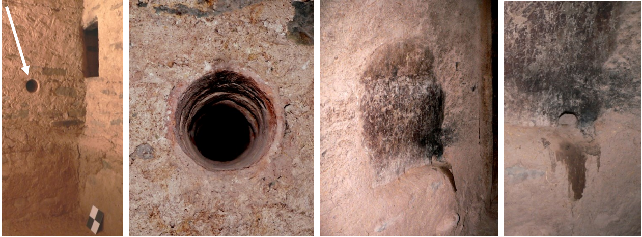
Figs. 17+18 Earthenware pipe of around 10cm diameter in the 40cm thick hammam wall
