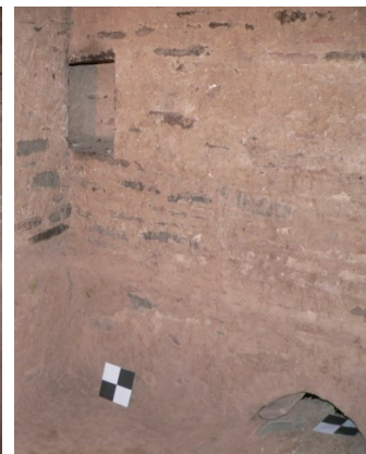
Fig. 8+9 Two different niches and a small arched wall penetration, probably for the heating system
